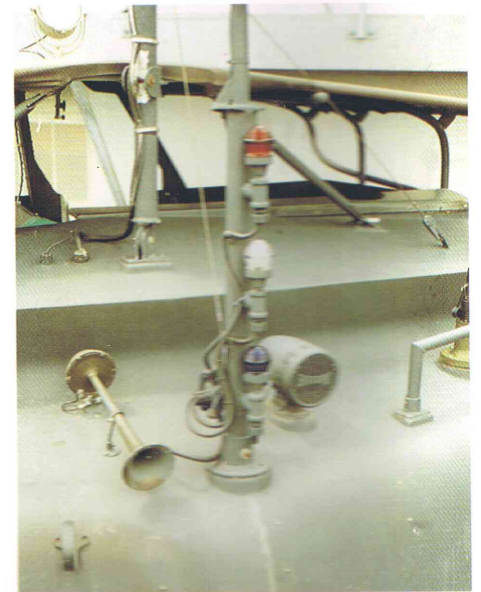
Fig.7 The siren, horn and forward light pole on the front of the charthouse.
